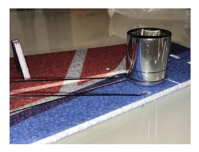
Just like the aileron bracing, it is very important to use weight towards the wing tip while the carbon wing bracing is set up to keep the leading edge of the wing as straight as possible.
